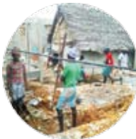
CLEARING OF LAND AND DIGGING OF 1 FOOT FOUNDATIONS
