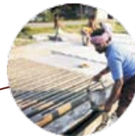
FABRICATION OF PRE-FAB RCC PILLARS AT A LOCAL YARD ENCOURAGING LOCAL ENTERPRISE
