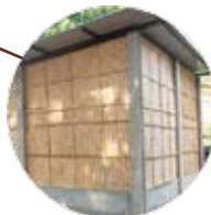
STRUCTURE WITH WALL AND ROOF
